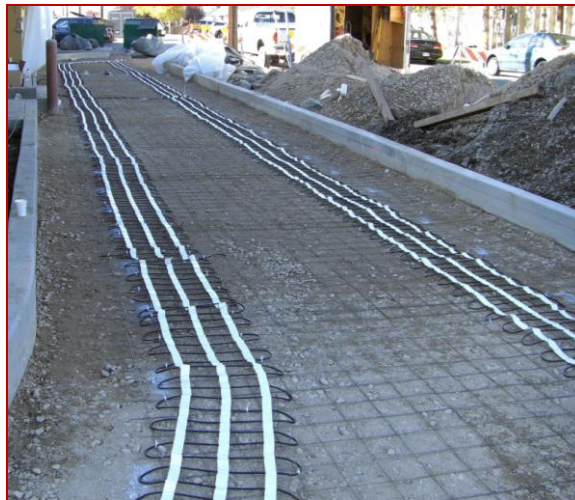
Heated tire track driveway being installed.
