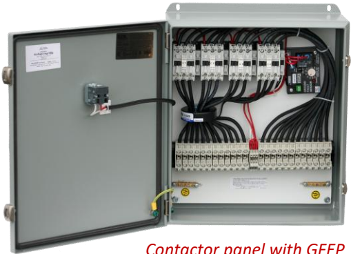
Contactor panel with GFEP
