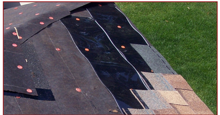
Heating element being installed under shingles.
