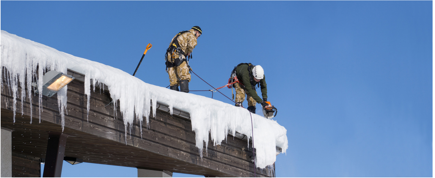
Shoveling and cutting down heavy, dangerous ice and icicles from the roof of a commercial facility.
