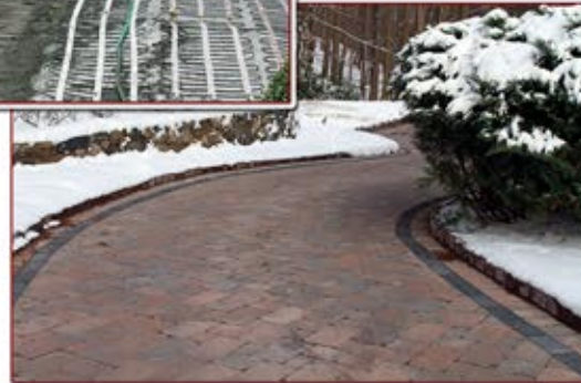
ProLine heating mats installed on sand base for heated paver driveway.
