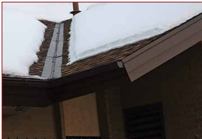
ProLine low-voltage roof heating element installed in roof valley.
