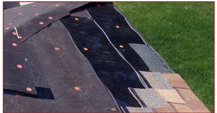
Heating element being installed under shingles.
