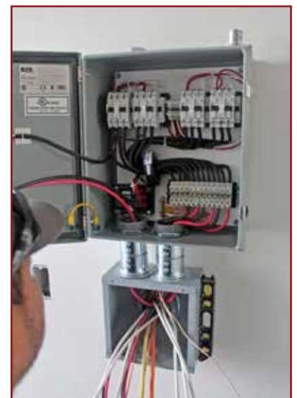
Contactor panel being installed.
