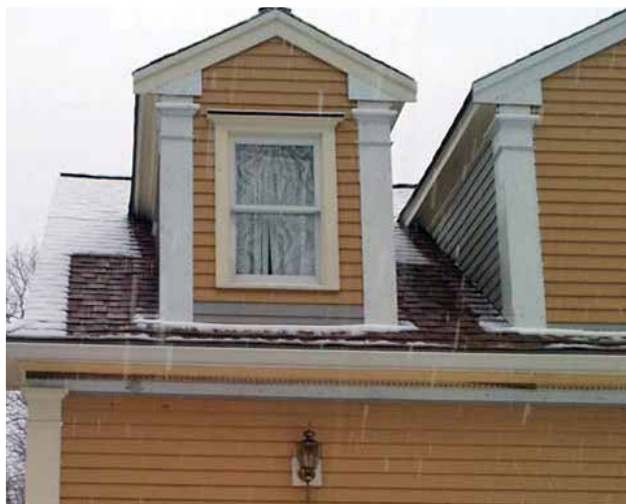
Roof deicing system heating roof edges.
