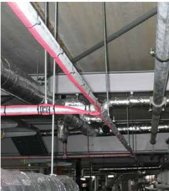
Pipe tracing system installed.
