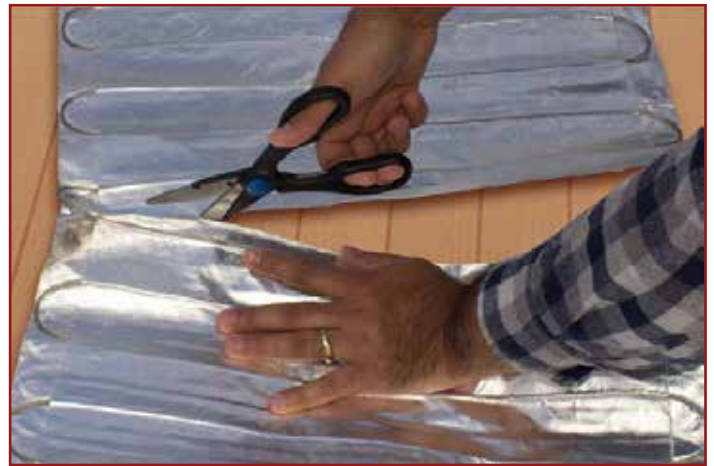
When cutting the mat to make turns (see illustration to the left), be sure to cut the mat only. DO NOT cut or damage the heat cable.
