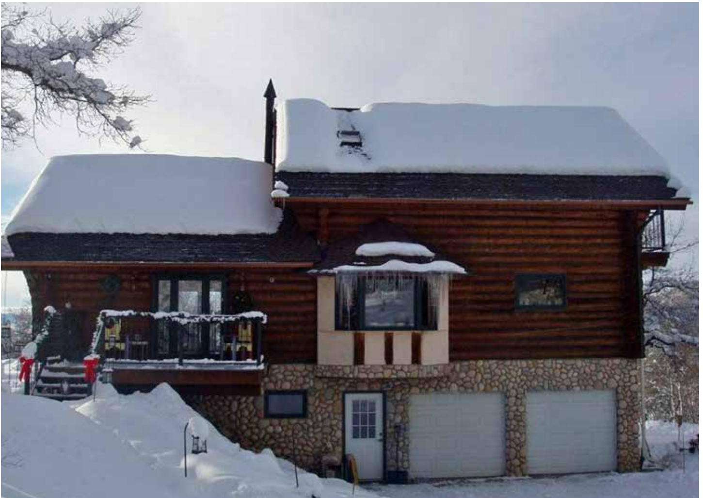
Mountain cabin with low-voltage roof deicing system installed at the roof edges.
