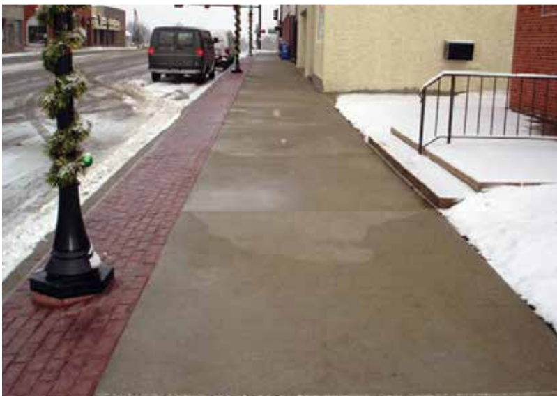
ProLine heat cable embedded in city sidewalks.
