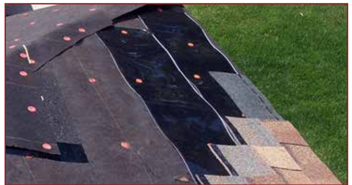
Heating element being installed under shingles.
