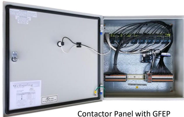
Contactor Panel with GFP
