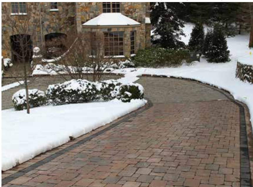
Snow melting system installed in paver driveway.
