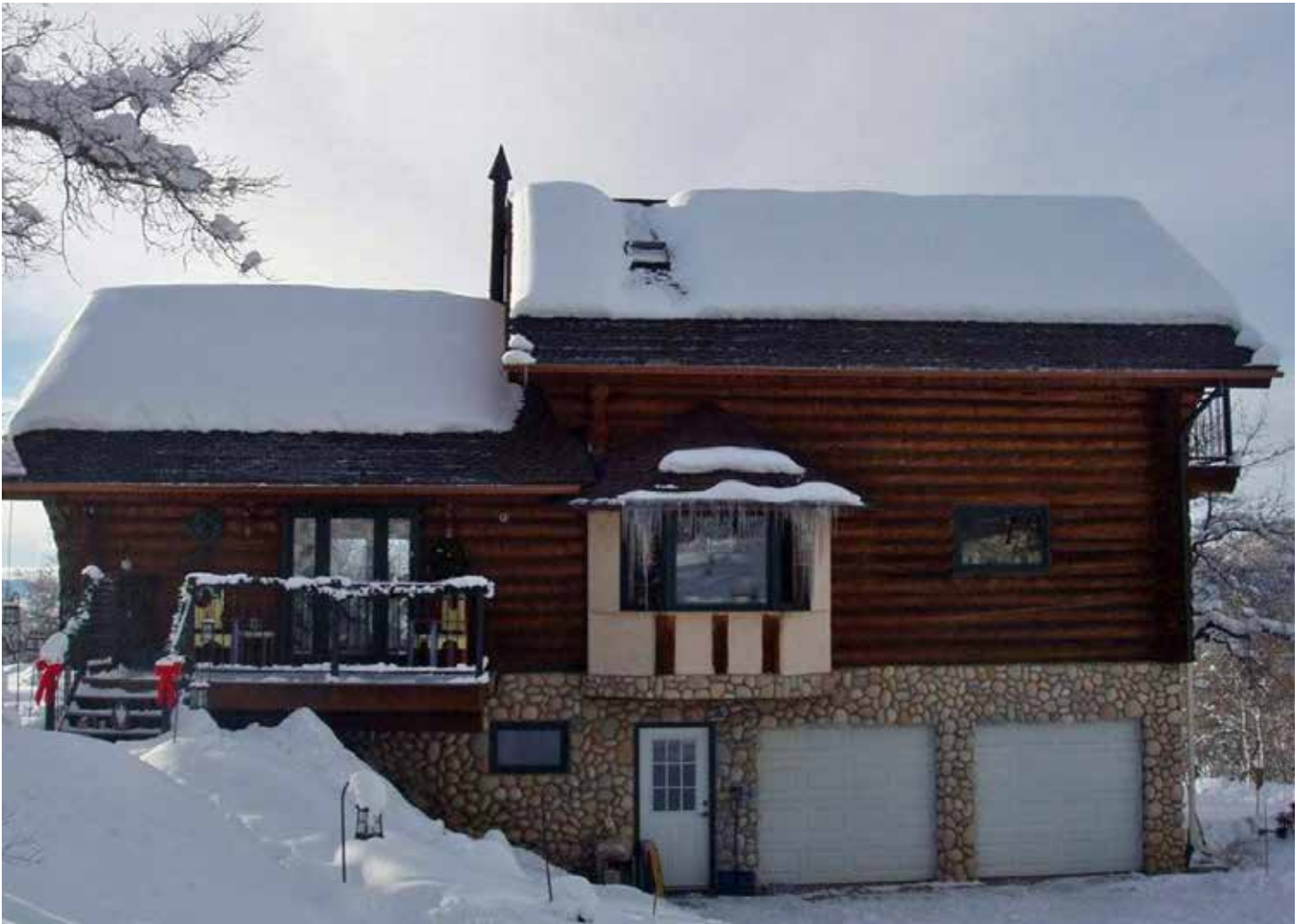
Mountain cabin with low-voltage roof deicing system installed along the roof edges.
