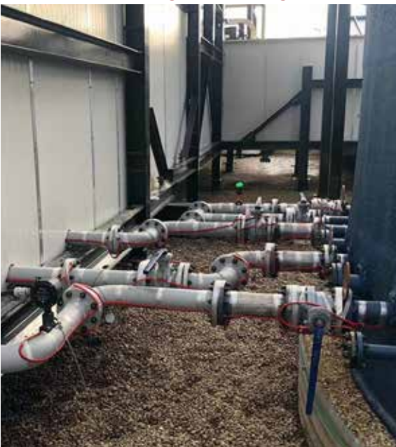
Pipe tracing system installed.
