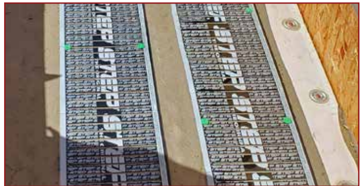
Heating element being installed under a metal roof at a public library.
