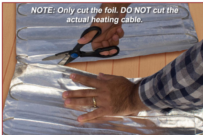
FoilHeat mats can be easily cut on site. (Depending on your heating requirement, FoilHeat is available in 120 and 240 volts at 12 watts per square feet.)
