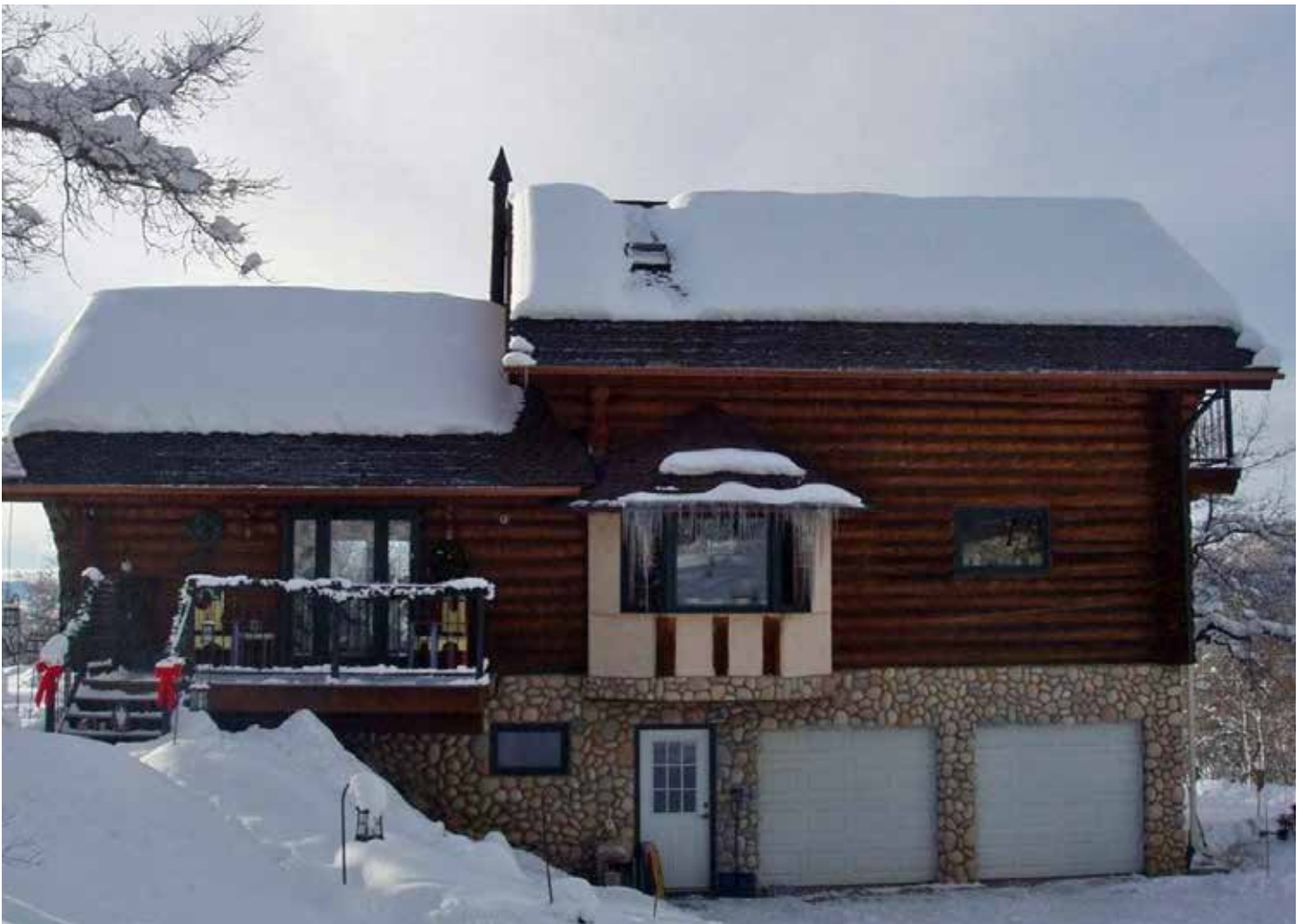
Mountain cabin with low-voltage roof de-icing system installed along the roof edges.
