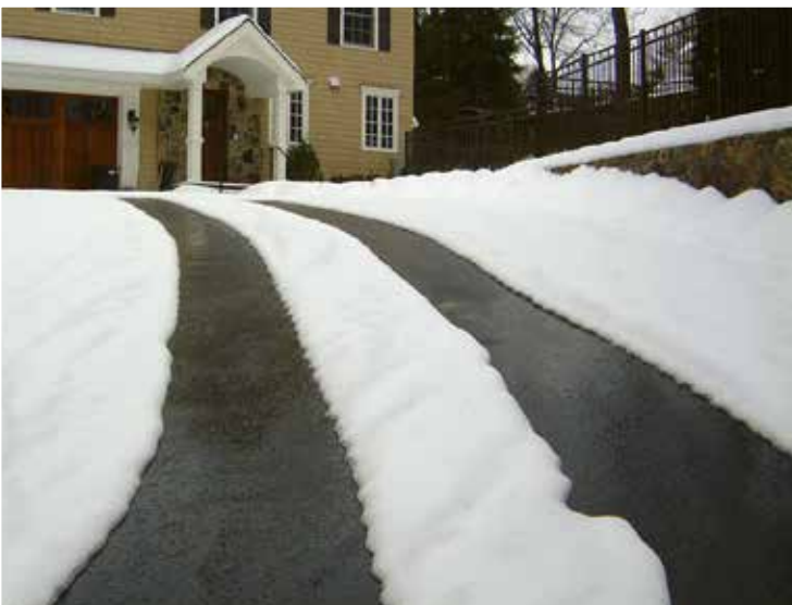
Heated tire tracks in asphalt driveway.
