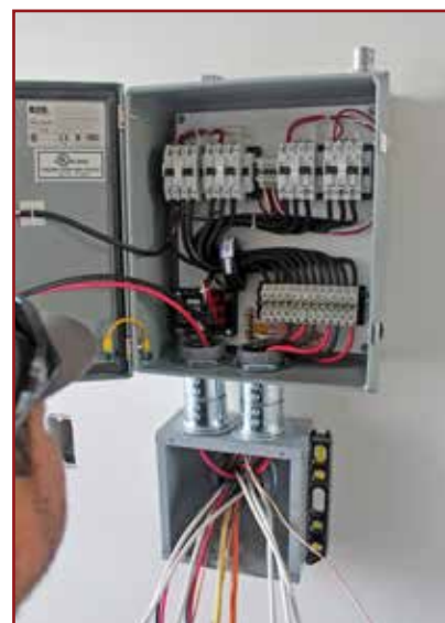
Contactor panel being installed.
