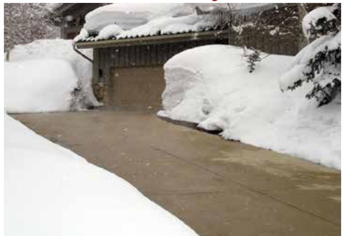
Radiant heated driveway.
