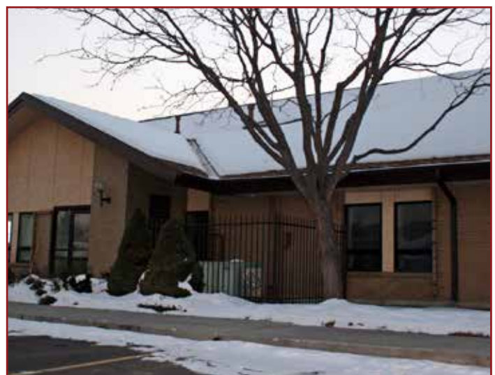
Commercial offices with the low-voltage roof heating system installed to heat the roof valleys and along the roof edges.
