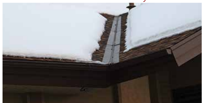
ProLine low-voltage roof de-icing system heating roof valley and edge.
