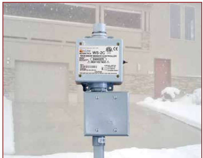
Example of a ProLine aerial-mount snow sensor and junction box.
