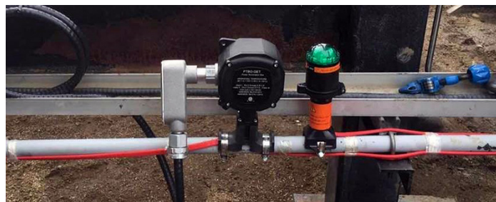
ProLine PTBO power connection kit and lighted end seal installed in industrial pipe trace application.
