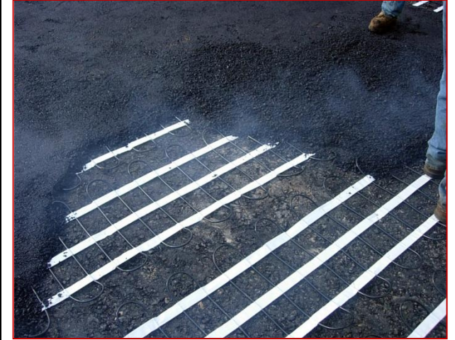
ProLine snow melting cable and mats are designed to withstand the extreme temperature of hot asphalt applications.
