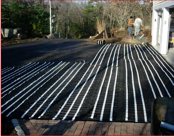
ProLine snow melting mats being installed for heated asphalt driveway.
