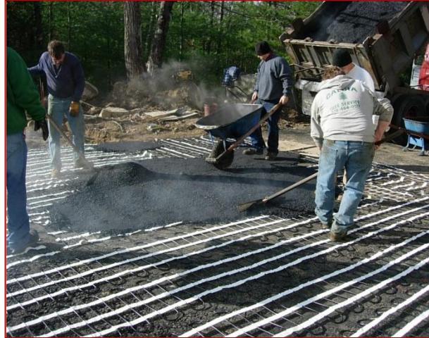
Hot asphalt being applied over ProLine snow melting mats.
