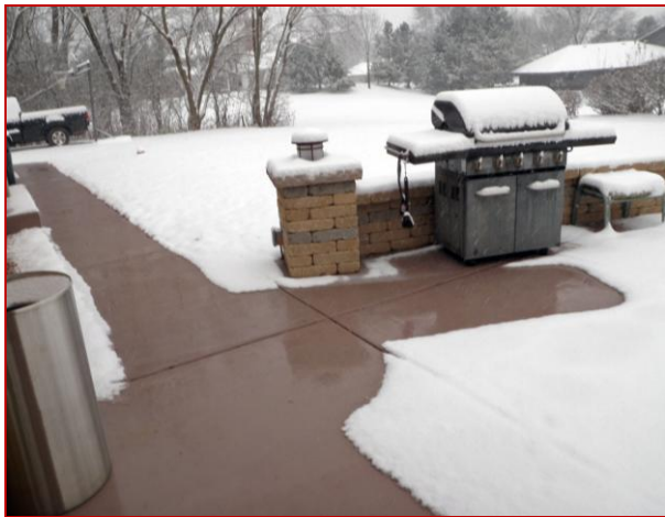
ProLine-heated concrete patio and sidewalks.
