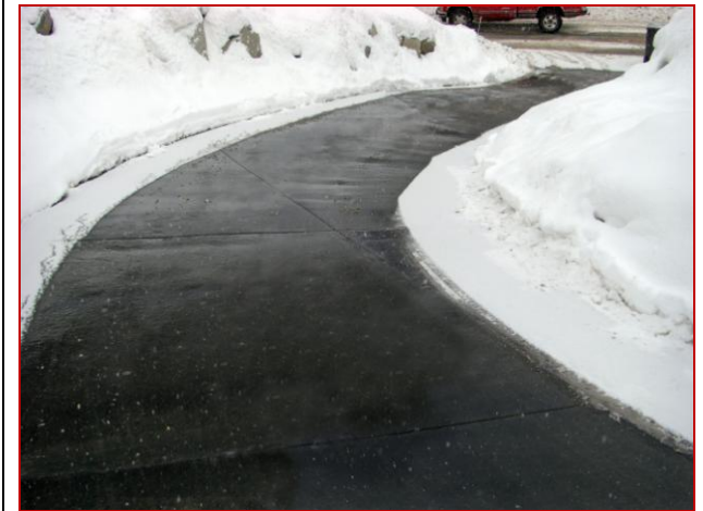
ProLine heated concrete driveway.
