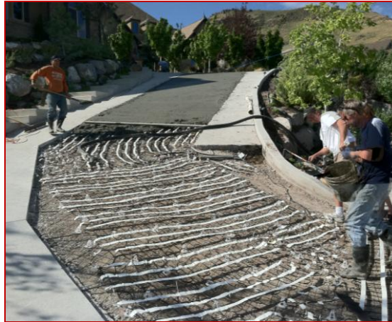
Pouring concrete over ProLine heat cable and remesh.
