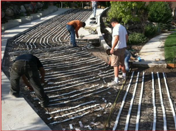
Laying out the ProLine heating mats.
