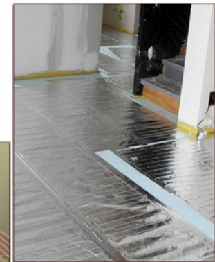
FoilHeat system being installed (above), and floor heating mats installed (left).
