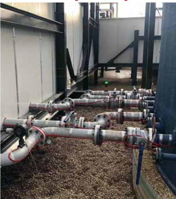
Pipe tracing system installed.
