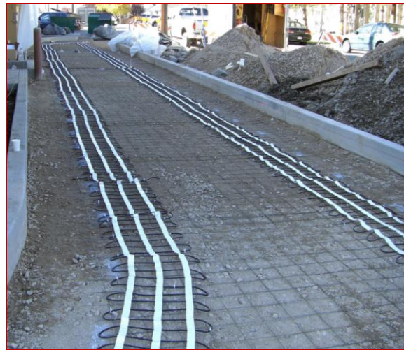
Heated tire track driveway being installed.
