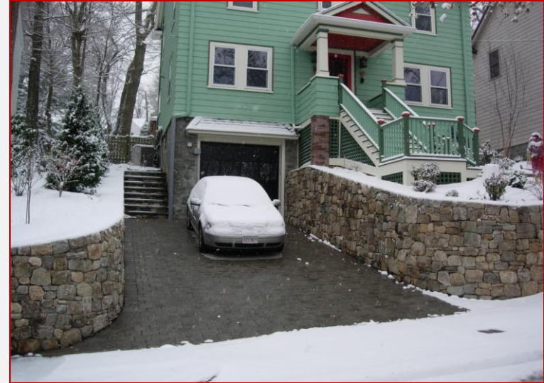
AFTER: ProLine paver heated driveway in operation.
