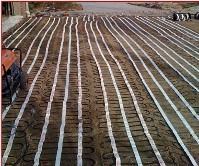
BEFORE: ProLine snow melting mats being installed.
