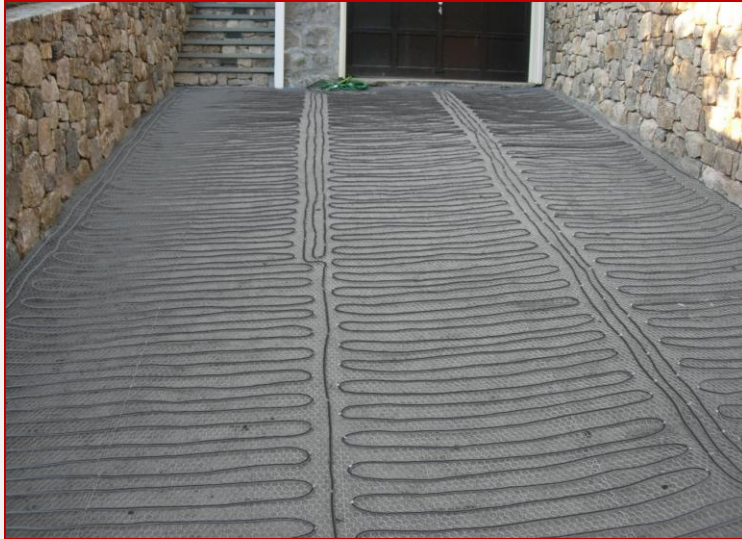
BEFORE: ProLine heat cable being installed under paver driveway.
