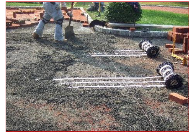
Installing ProLine snow melting mats for heated paver driveway.
